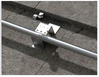
Use self-tapper screws or included hardware to mount conduit straps or junction box bracket. Refer to the NEC for required conduit spacing.
