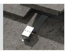
**3**Lower lifted tile and adjust adjacent tiles if any tile spacing has been disturbed by the installation.
