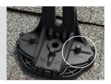
3 Insert the lag screw through the center hole into the pilot hole.
