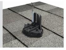
**4**Drive the lag until the InstaFlash is fully seated to the roof.
