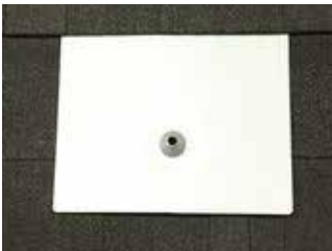
NOT OK Flashing must NOT extend beyond the bottom of the first shingle course.
