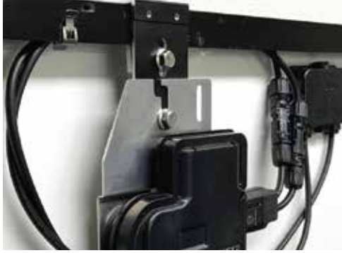
Slightly braid the module wires and connect them to the micro-inverter or optimizer. Secure wires to module frame using stainless steel wire clips.
