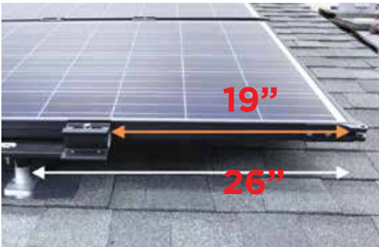
Double Assembly increases cantilever.
