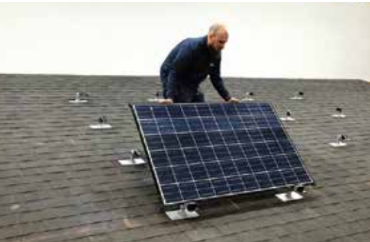
First row of Mounts facing down the roof, set module onto Mount.
