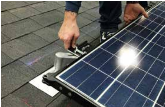
Rotate the second row of Mounts onto module.
