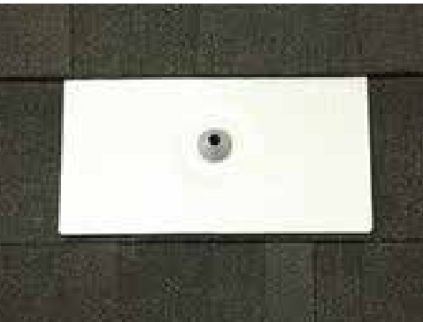
OK Flashing extends fully under two courses of shingles.
