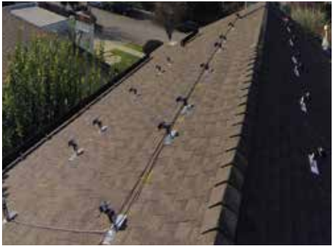
Home run and jumper wires should be run prior to module installation. A/C conduit and combiner boxes should be complete.
