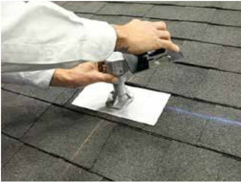
Place Mount on Base and spin clockwise.
