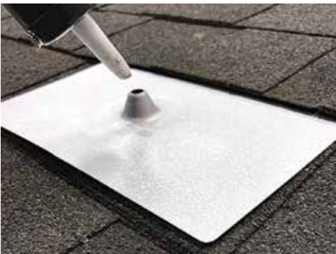
Filling volcano with approved sealant is recommended.
