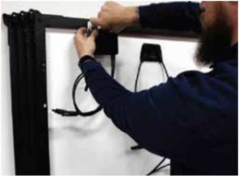
Install MLPE Bracket on module. Micro-inverter or optimizer. Wire management should be done on the ground before module installation.
