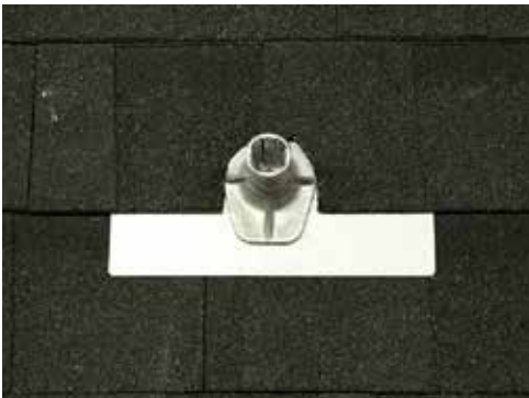
OK Notching shingle around base.
