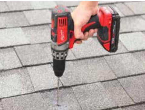
Drill pilot hole into rafter with a 7/32" drill bit.
