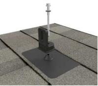
**4.** Drive lag to required depth. Attach rail per rail manufacturer's instructions.
