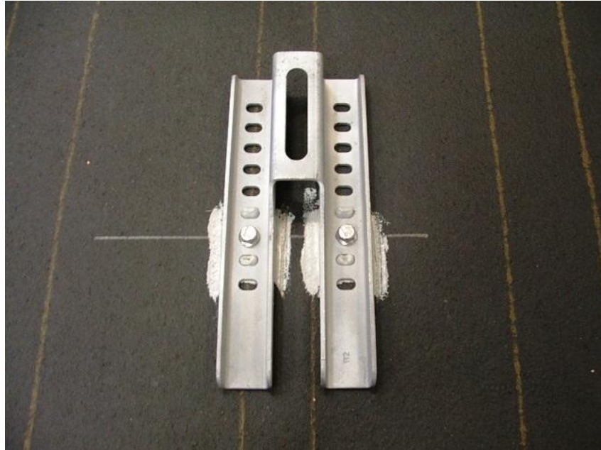
Photograph No.1 Tile Sled Mounted on Roof Deck No.1
